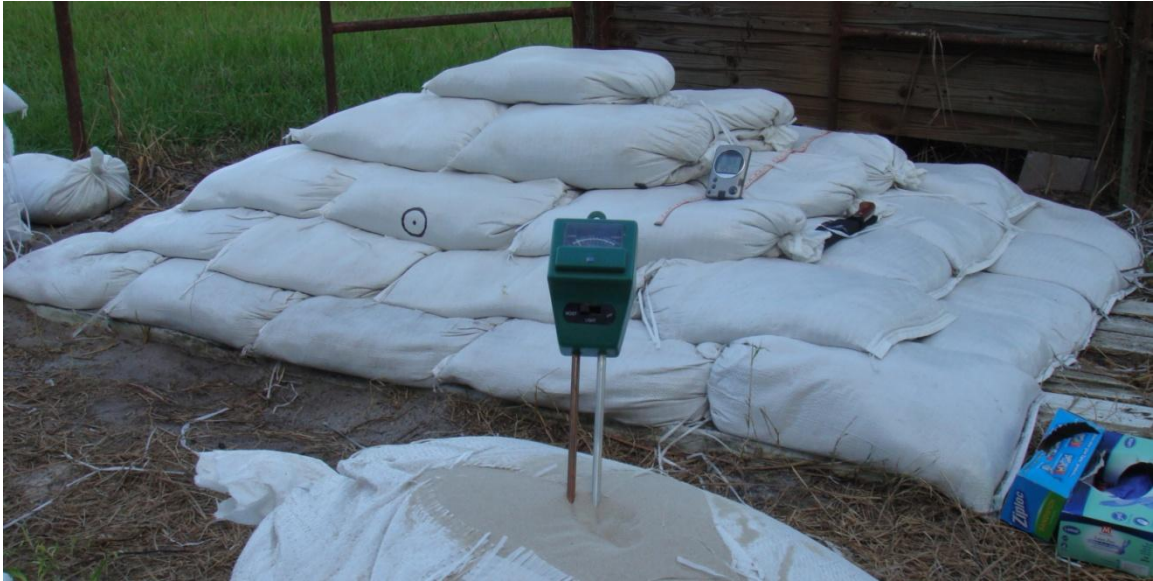
Figure 28 Assembly of the Sandbag Barrier
